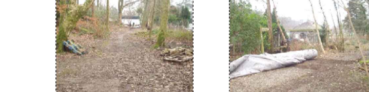
Photo 1 - Use of wire mesh prior to the commencement of works. Photo 2 - Laying of Fibres F4M non-woven geotextile material onto existing subgrade.
