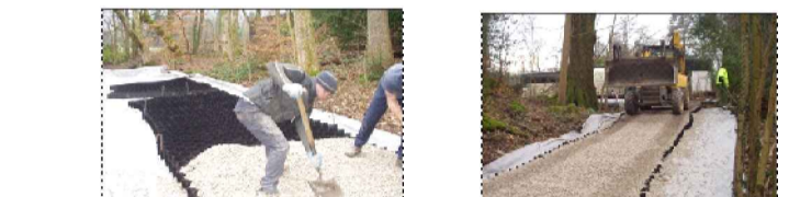
Photo 1 - Ultrasonic welding of the Cellweb system. Photo 2 - Final cellular confinement system (polyweld) in situ aggregate in the fill.
